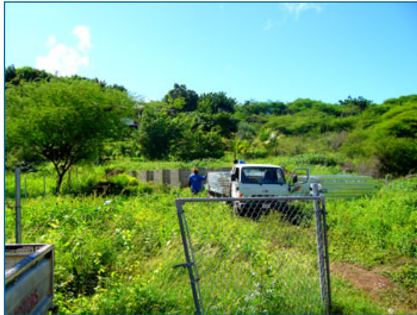
Delivery of the steel framework
